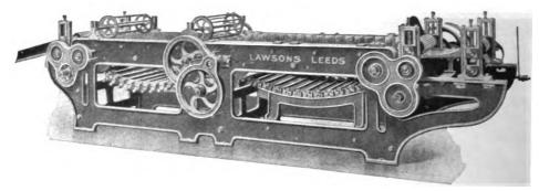
Fig. 11.—Good's Hackling and Spreading Machine.
