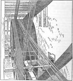
Fig. 6.—Rope Race of a Lancashire Cotton-Spinning Mill, with 38 Lambeth Cotton Driving Ropes, 11 in. diameter; engine, 1700 H.P.
